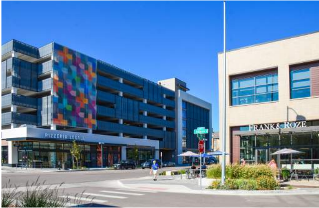
(Left) Example of exposed parking structure in pedestrian-oriented urban neighborhood that utilizes a series of decorative panels, feature walls, and changes in facade plane to create a visually attractive parking structure. (Right). Parking structure facade is organized compositionally like a building with a distinct base, fenestrations, and a series of features walls of varying materials, one of which was use for signage.
