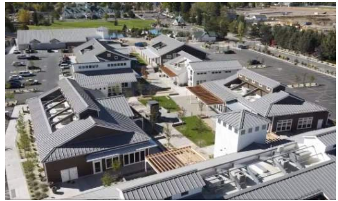
(Left). Freestanding retail frontage uses varying parapet heights to screen mechanical and utility equipment on the roof. (Right) Retail village with farm-style shed roofs with clerestory roof projections create voids within roof forms to discretely hide mechanical and utility equipment
