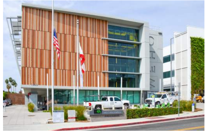
(Left) Example of exposed parking structure in pedestrian-oriented urban neighborhood that utilizes a series of decorative panels, feature walls, and changes in facade plane to create a visually attractive parking structure. (Right). Parking structure facade is organized compositionally like a building with a distinct base, fenestrations, and a series of features walls of varying materials, one of which was use for signage.
