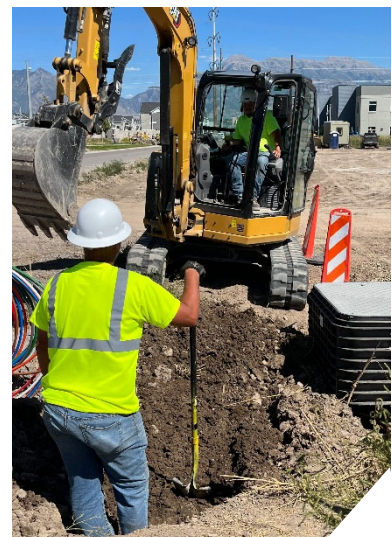
FIBER VAULT INSTALLATION
