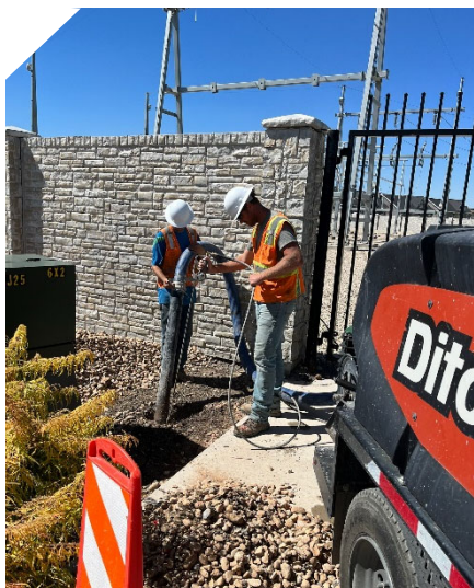
VAC UTILITY EXCAVATION
