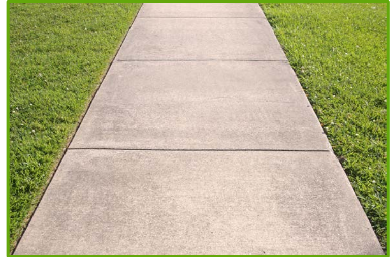
Infrastructure Improvements & Maintenance
