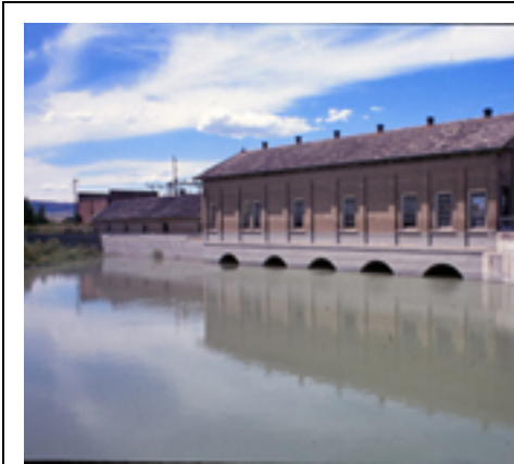
Utah Lake Pumping Plant viewed from the inlet side. Circa. 1990
