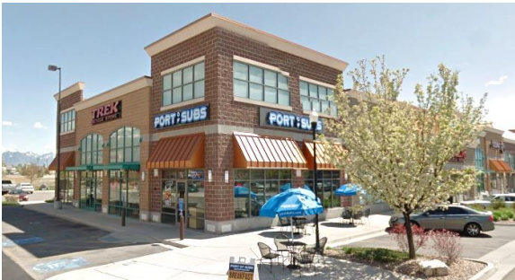
Figure 5. Retail building with clear windows on the ground floor exceeding 50% of the front façade.
