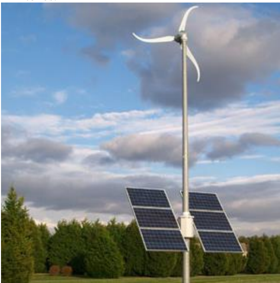
Figure 2. Hybrid wind and solar energy facility
