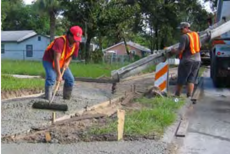
Construction workers pour concrete as part of a sidewalk improvement project
