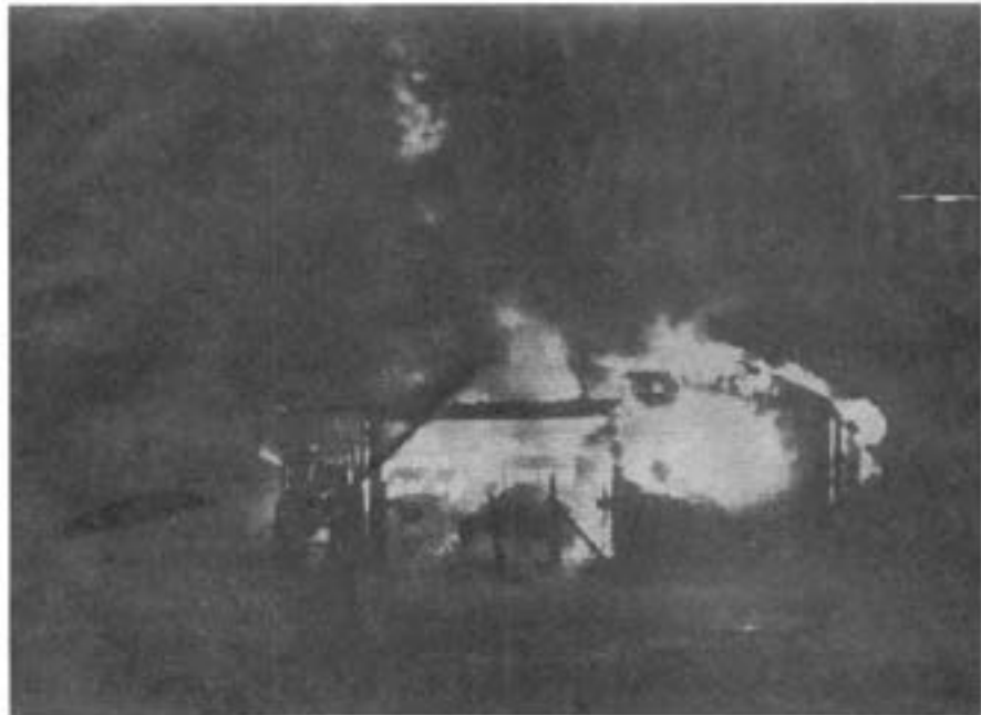
Figure 18 Fire at Camp Williams fire department
