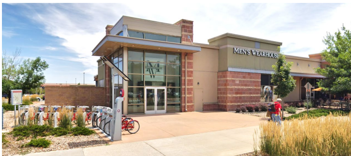
Figure 82. Retail building provides public building entrances facing the public sidewalk.
