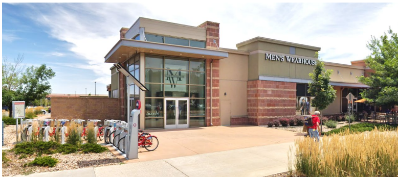
Figure 105. Retail building provides public building entrances facing the public sidewalk.
