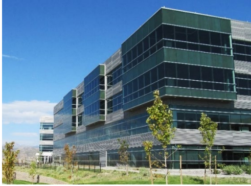
Figure 108 – Metal used is of a high grade and provides an architectural quality to the building.
