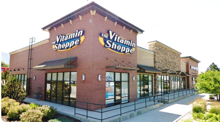
Figure 110. Stucco is only applied to recessed and secondary wall areas, and the hierarchal features use brick and rock.
