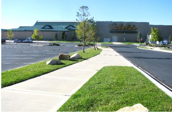
Figure 166. Parking lot pedestrian walkway with pockets of landscaping.
