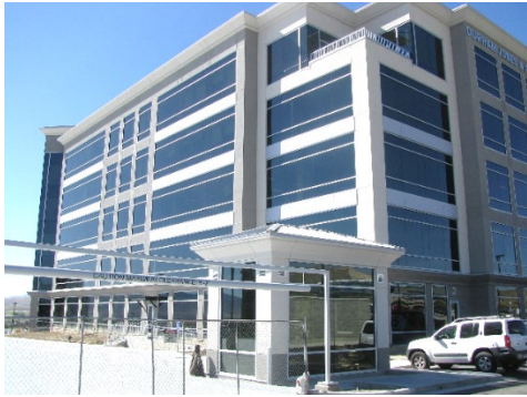
Figure 176. Parking structure stairway is enclosed with the use of materials to match the principal structure.
