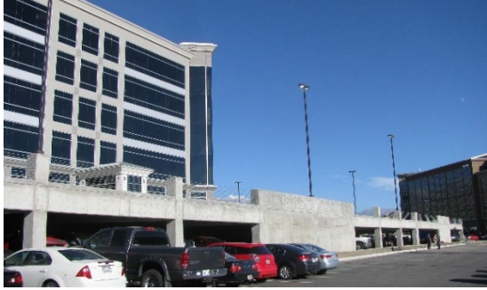
Figure 175. The parking structure facade exhibits variations with the use of embossed concrete walls and the use of pillars and cable.
