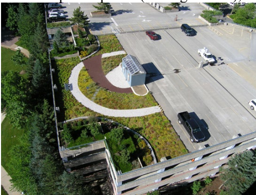
Figure 177 – Top deck of a parking structure with large elaborate landscaped area and landscaping around the base of the structure.
