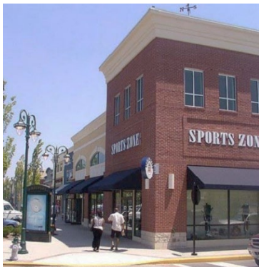
Figure 117. The first floor facing the street includes large clear glass windows.
