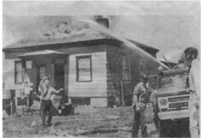
Figure 41 Roof fire at Lafayette Jones
