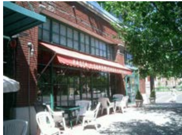
Example of Glass in Transom Windows
