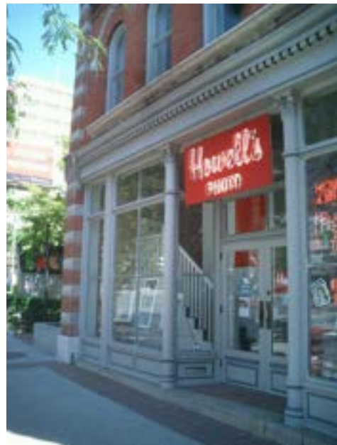
Original Recessed Entrance has been Maintained
