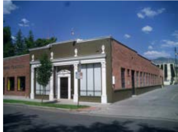
Unfortunate Remodeling that Superimposes a Fake "Historic Style" on an Existing Building
