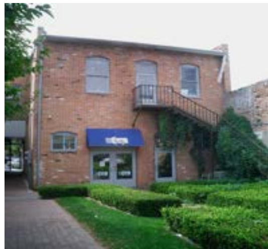
Awning Identifies a Public Door in this Rear-facing Facade
