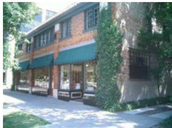
Good Remodeling that Respects the Existing Building and Uses Clear Glass Between Structural Piers
