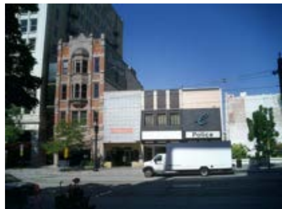
Second-story Window Openings have been Covered by Inappropriate Remodeling
