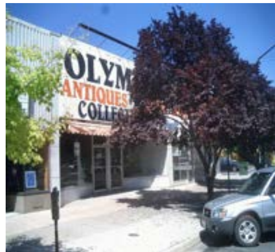
Sign Overpowers the Façade and Obscures Building Features
