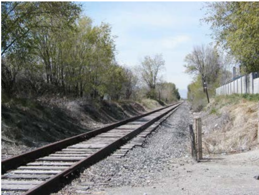
Existing Rail Lines Provide a Multi-Purpose Trail Opportunity
