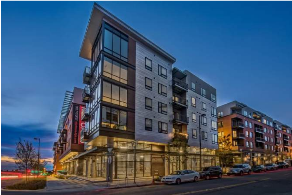
Figure 5. The ground floor for mixed use buildings should have greater height and massing, and larger windows proportional to the use.
