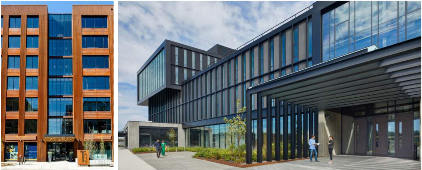
(Left). Building uses a central recessed element to create articulation in the facade combined with more glass, awning, and signage to identify building entrance. (Right). Increase fenestration, material changes, and a projecting trellis structure creates a portal to highlight the building entrance and provides articulation in the building facade.
