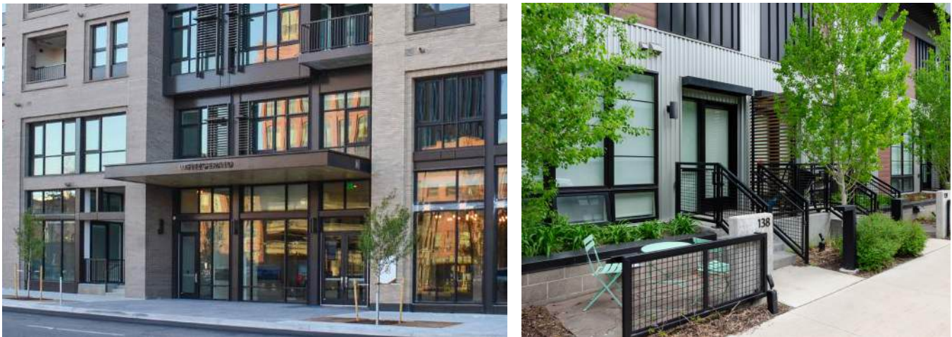
(Left). Lobby entrance facing the street is recessed and articulated with more glass, awning, signage, and lighting to clearly distinguish within the architectural treatment of the base. (Right). Ground floor unit is elevated slightly above the street but has direct access via a stoop to the street as well as from a corridor internal to the building access from a shared building lobby.
