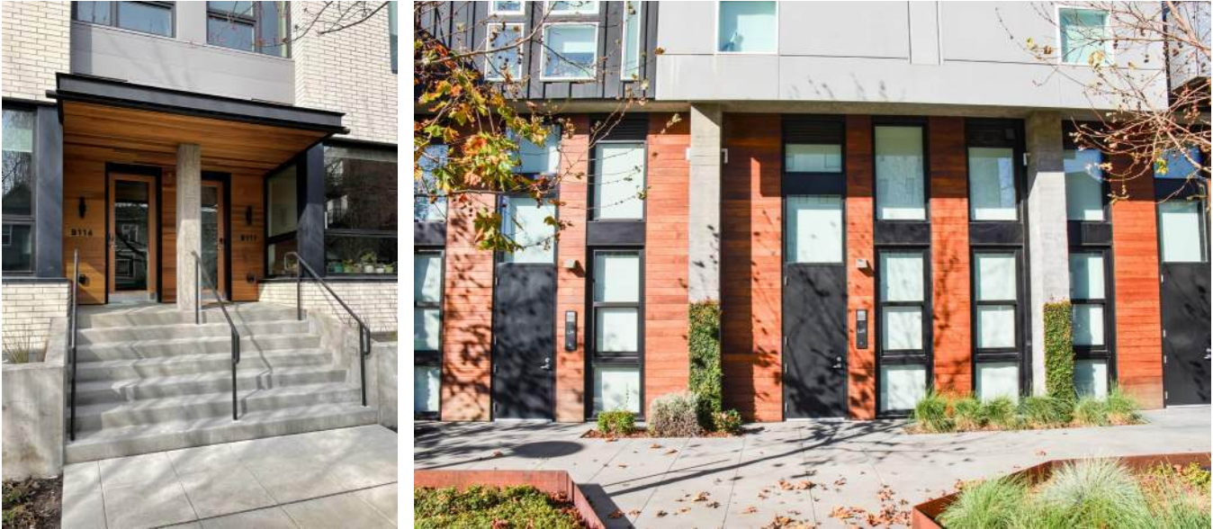
(Left). Townhome style ground floor units include stoops and raised planters to create privacy through a grade separated entrance in the base of a multi-family building. (Right). These townhome style units ground floor entrances that orient to a publicly accessible open space.
