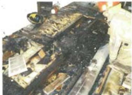
Figure 122 Tim Hunt views the damage
