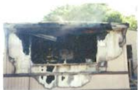
Figure 113 Kitchen of Trailer house
