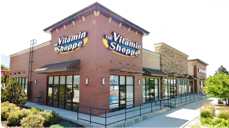
Figure 128. Stucco is only applied to recessed and secondary wall areas, and the hierarchical features use brick and rock.
