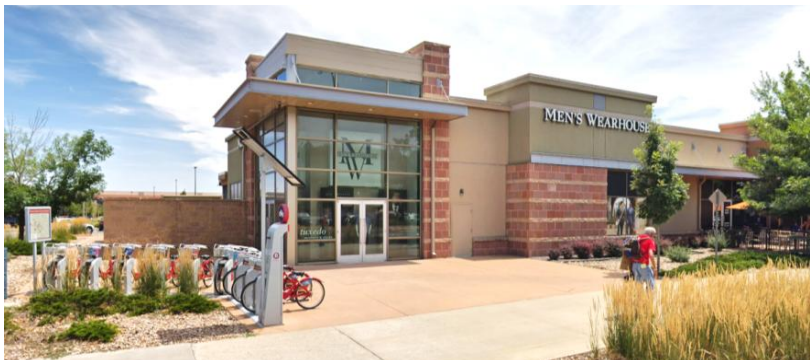
Figure 123. Retail building provides public building entrances facing the public sidewalk.
