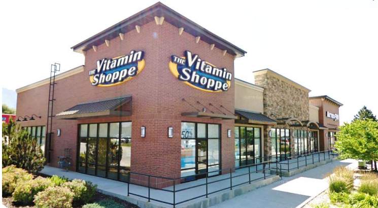
Figure 68. Stucco is only applied to recessed and secondary wall areas, and the hierarchal features use brick and rock.
