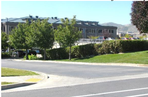
Figure 174. Parking structure built into the slope with low visibility from the street.
