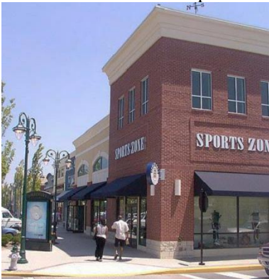
Figure 95. The first floor facing the street includes large clear glass windows.
