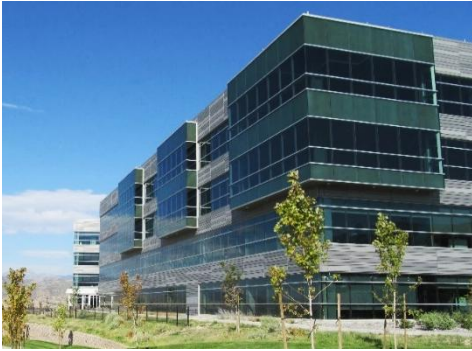
Figure 53 – Metal used is of a high grade and provides an architectural quality to the building.
