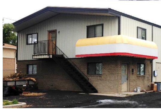
Figure 109 – Metal used is an industrial grade and has the appearance of standing seam metal which detracts from the architectural quality of the building.
