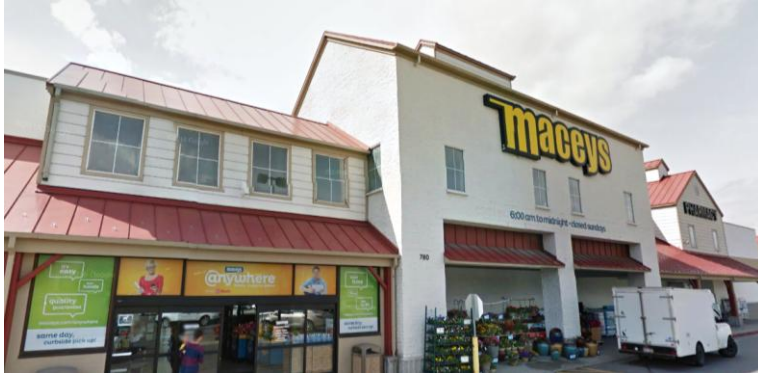
Figure 28. Existing building includes pitched roofs with cupolas which is characteristic of the historic Lehi Roller Mills.
