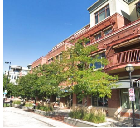
Figure 6 – Appropriate building that utilizes articulations and balconies to break up the facade and reduce the perceived scale.
