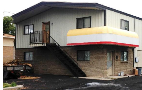
Figure 127 – Metal used is an industrial grade and has the appearance of standing seam metal which detracts from the architectural quality of the building.
