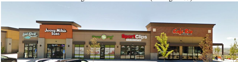
Figure 63. Two hierarchal building features are included on this building for separate entrances.
