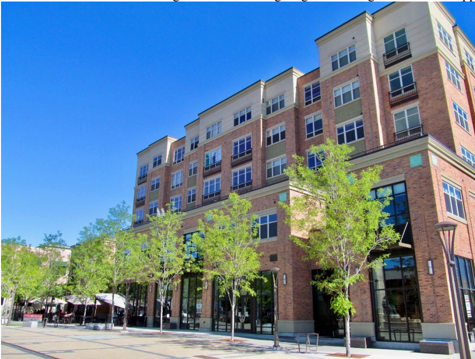
Figure 6. The ground floor includes large windows and has greater mass and height than the upper floors of the building.
