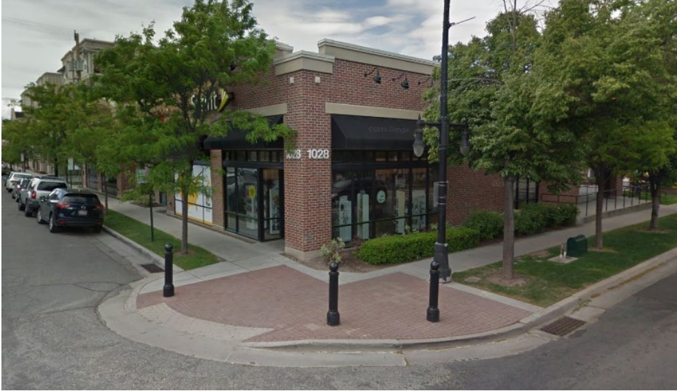
Figure 10. Bulb-out provides traffic calming, increases visibility to drivers, and shortens pedestrian street crossing distances.
