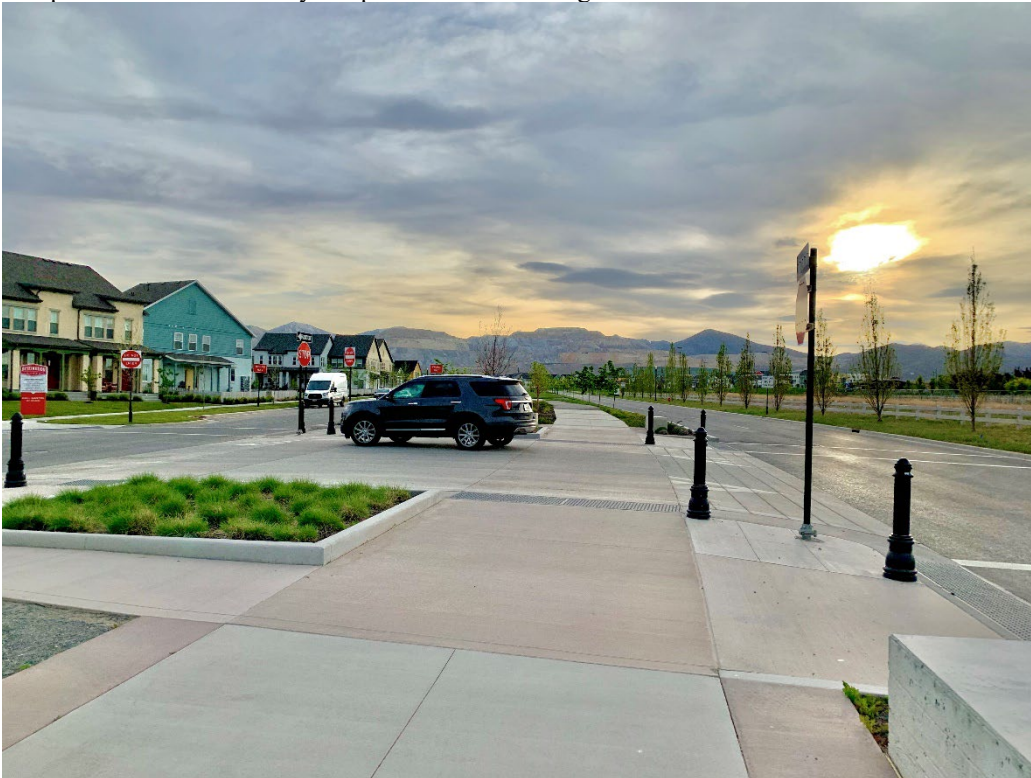
Figure 15. The trail and sidewalk run continuously and built with consistent materials whereas vehicular traffic must ramp up to cross the bike path and sidewalk. This slows traffic at a bike and pedestrian conflict point and indicates to drivers that they are entering a bike and pedestrian space.
