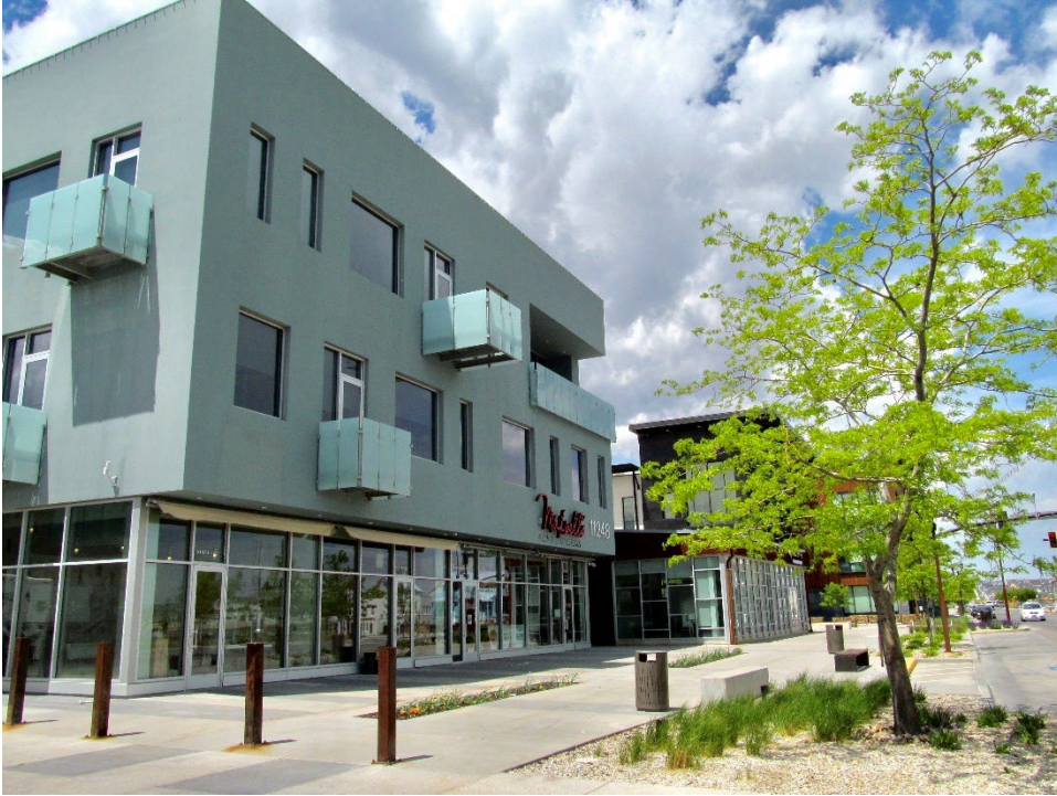
Figure 5. Retail building with clear windows on the ground floor exceeding 50% of the front façade.
