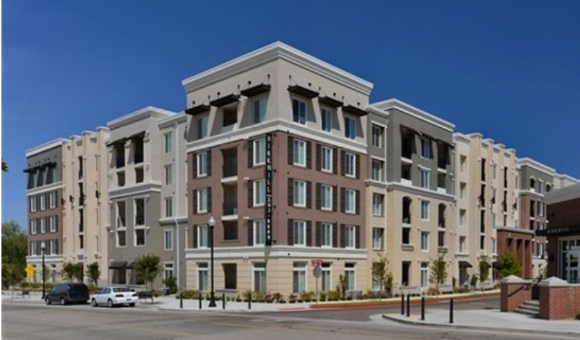
Figure 3. The apartment building includes a flat roof design with varying parapet heights and an architectural hierarchy to the street corner.
