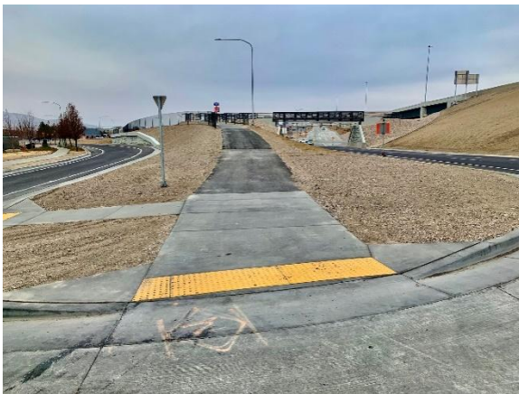
Figure 4. The ramp and truncated dome width match the trail width.
